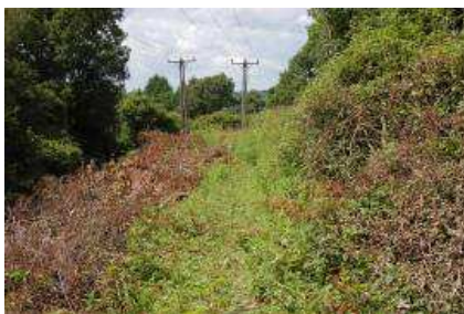
Figure 1: Telephone wire Wayleaf (Public Footpath) with clearing of scrub currently in progress.
